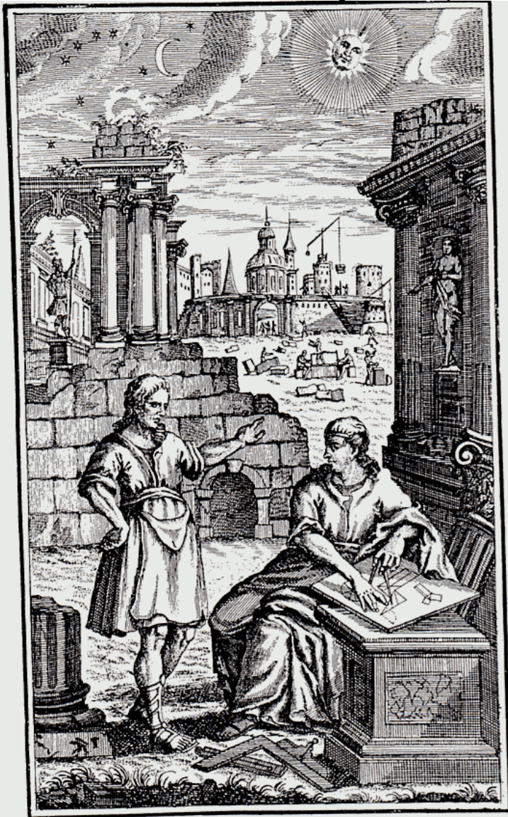
(1738 German Drawing depicting workmen using the 47 th problem)
